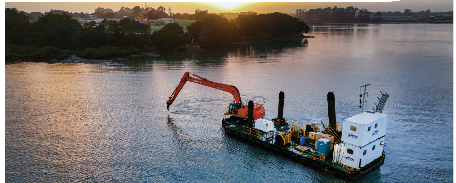
Pictured above: A combi barge – combination of a barge and excavator – is used to construct a tunnel boring machine retrieval pit in the Waiuku channel. This is an essential part of the Clarks Beach outfall pipe project.
