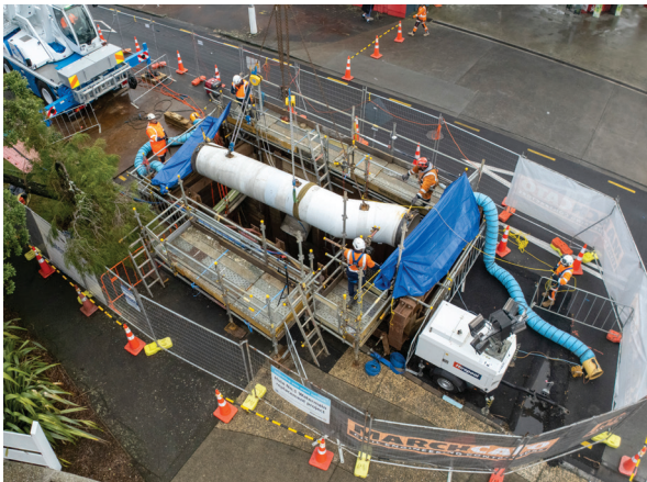
One of the final sections of the Huia 1 replacement pipeline being lowered in on Heaphy Street in Blockhouse Bay in April 2025.
