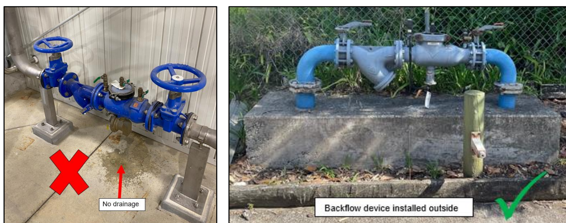
Figure 2.2: Example of a backflow device installed inside a building with no drainage, creating a flooding risk.
