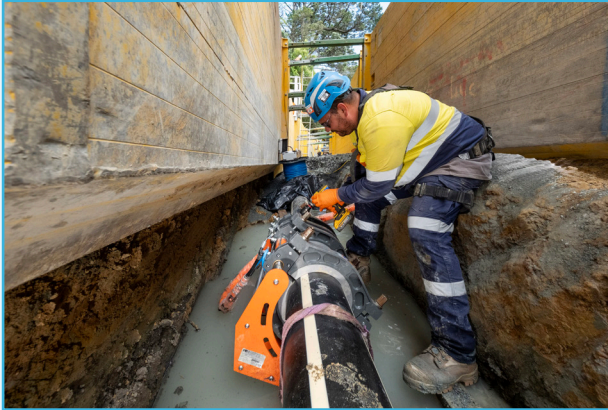
Installation of the water and wastewater pipeline via open trench along the Hibiscus Coast Highway.
