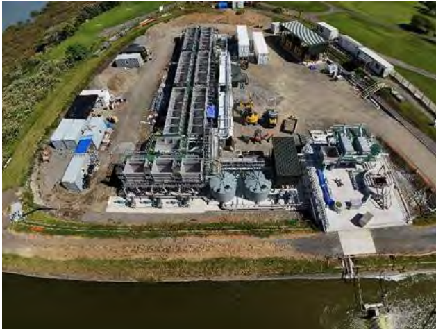
Upgrade at Clarks Beach WWTP site
