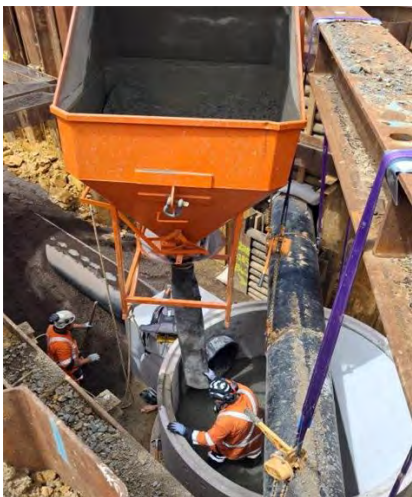
Pouring corbel for Rosedale Rising Main
