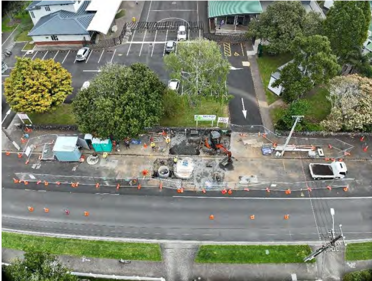
Installation of line valve and scour valve chambers on Richardson Rd.
