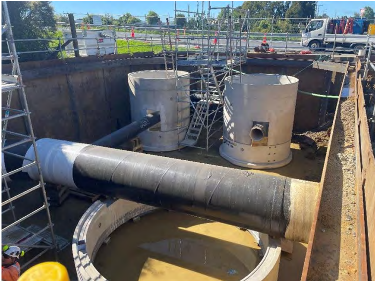
First half of the temporary shaft and layout incorporating new pipework
