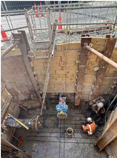
Location for new Line valve chamber
