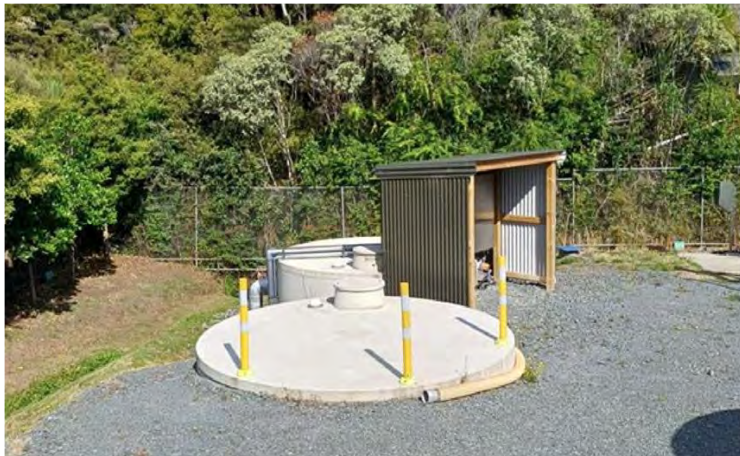
Reinstated WTP connection point to the new Snells gravity sewer
