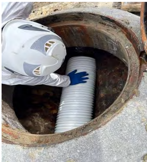
PVC Spiral wound relining of a 300mm gravity pipeline underway
