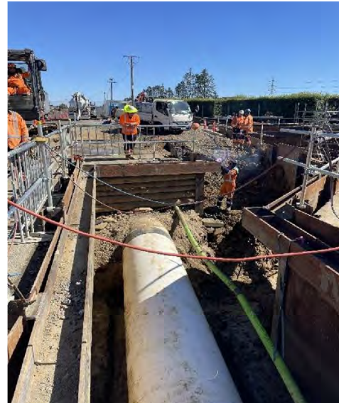
Start of the excavation for the second half of the shaft
