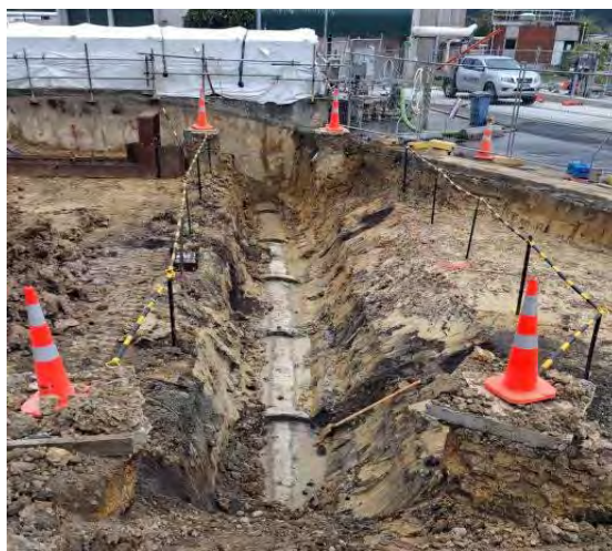
Wairau Valley Branch Sewer exposed for the start of confluence chamber construction
