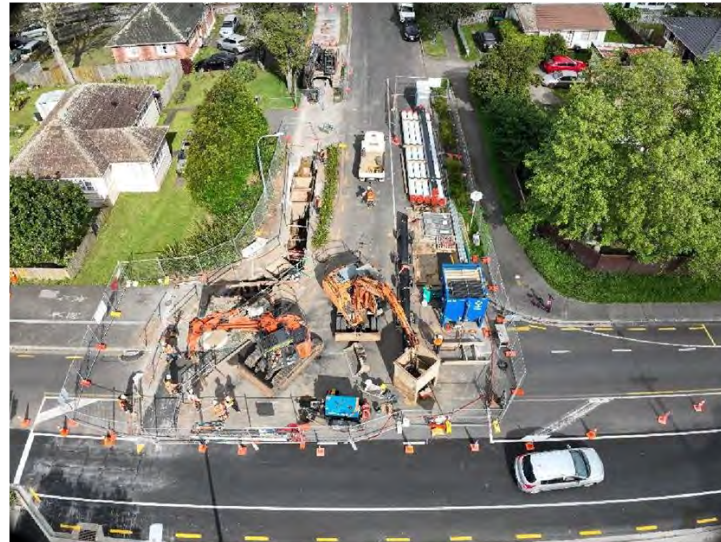
Pipelaying work at the corner of Memorial Ave and May Rd
