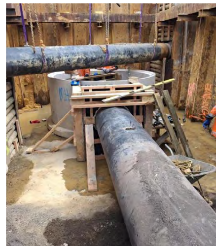
Rosedale Rising Main suspended during manhole construction
