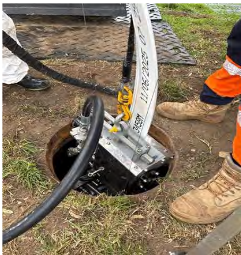
PVC Spiral wound relining of a 300mm gravity pipeline underway
