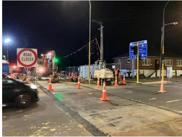
Night works for Dominion Rd crossing
