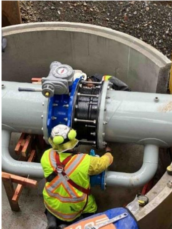
Construction of valve chamber on La Veta Ave
