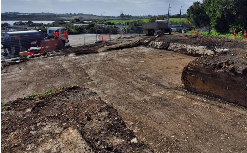
Confluence chamber reduced dig to prep for bore piling
