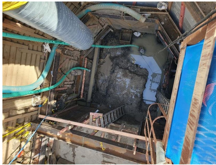
Excavation within the Victoria Street shaft
