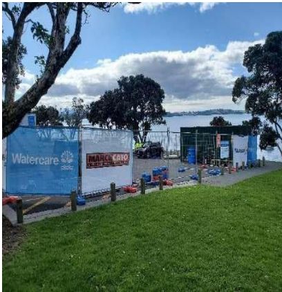
Saline Intrusion Rehab Site office
