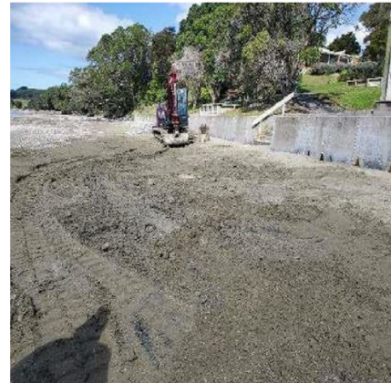
Algies Bay Collection Rehabilitation
