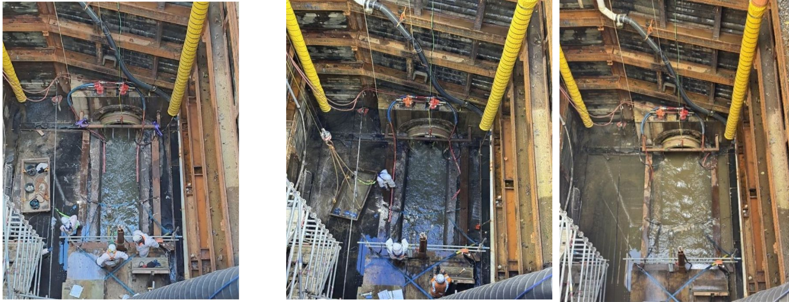
Recommencement of works following high sewer levels
