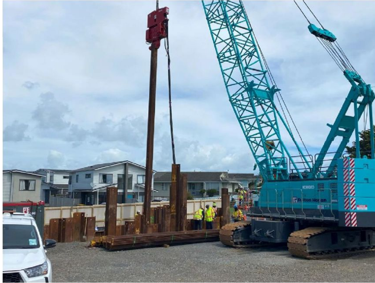
Pile Installation Wet Well & Inlet Manhole
