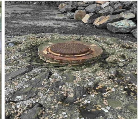
Typical Manhole to be replaced
