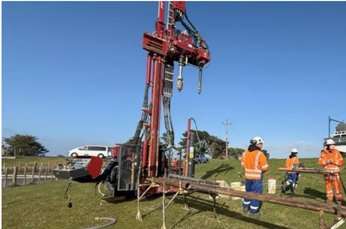
Boreholes undertaken at the Waiuku WWTP site
