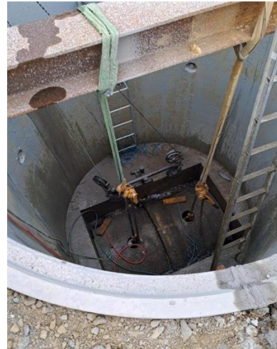
Wairau VBS in new manhole for lining
