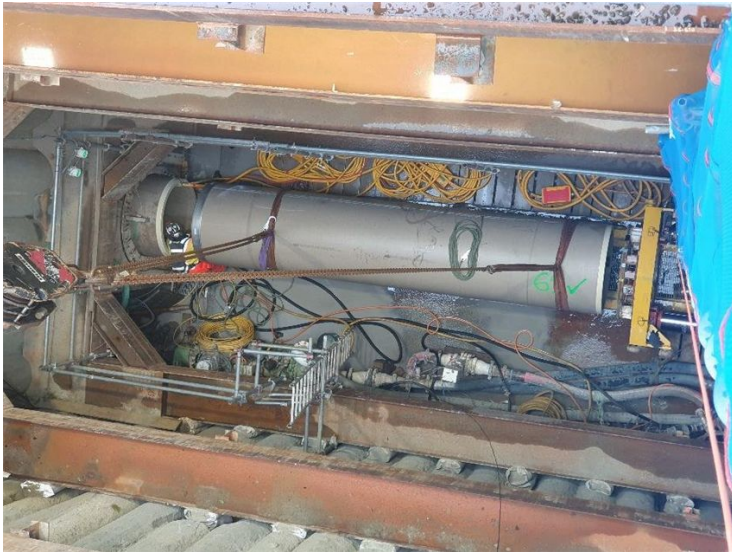
Pipe Jacking from Mayoral Drive shaft
