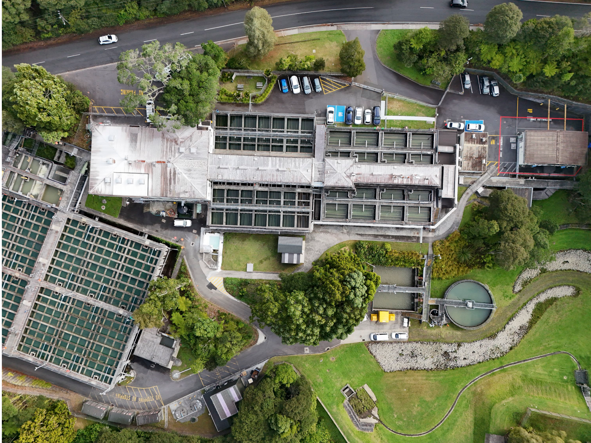
Image: Huia Treatment Plant.
