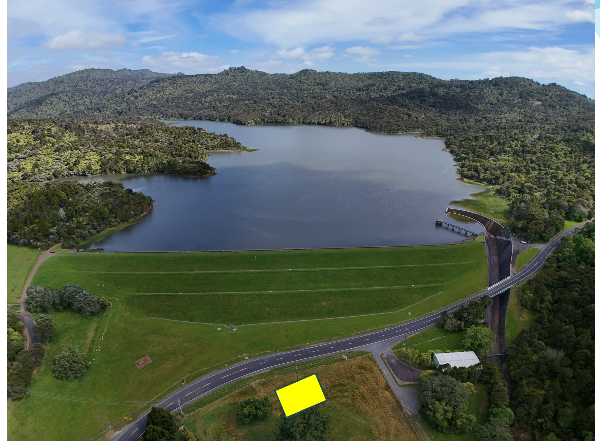
Image: Lower Nihotupu dam.
