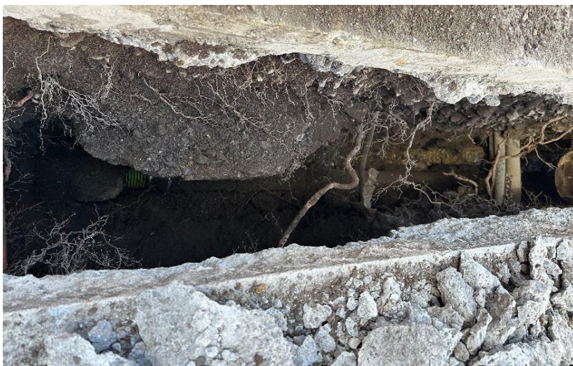
Figure 4-11: Previous investigation works to the south of Tree 8 showing minor roots in proposed footpath manhole connection location
