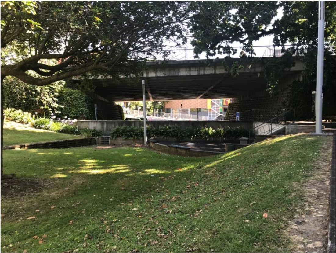
Figure 2-2: Detention Basin at Myers Park
