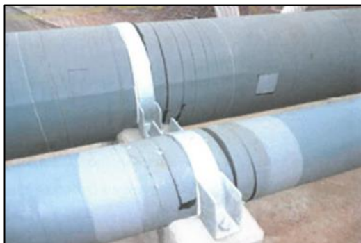
Figure 5: Example of hoop strapping installed on pipe bridge
