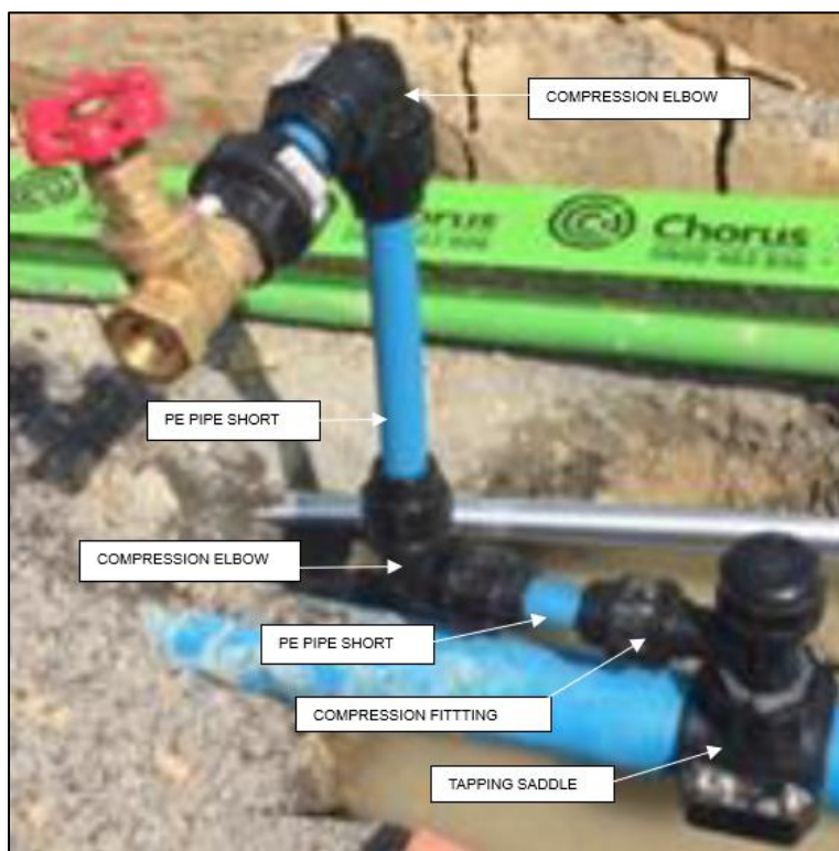
Figure 21: 1) Installation of a tapping band, compression couplers and gate valve.
