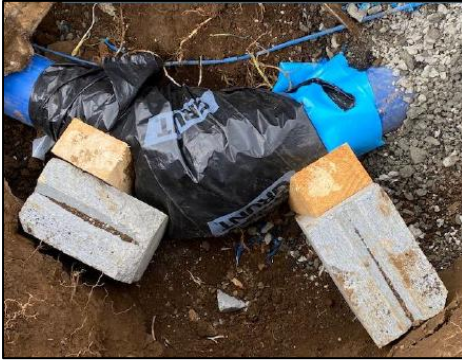
Figure 10: Example of kerb blocks being used for temporary support before casting in-situ concrete.
