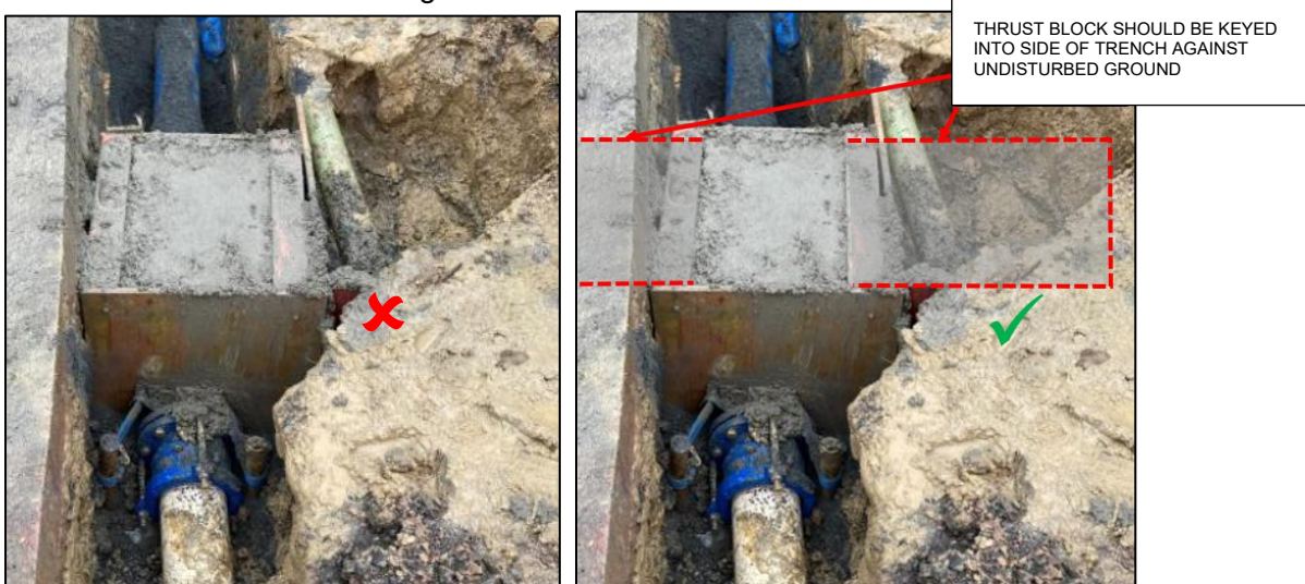
Figure 12: Example of incorrect installation, where concrete does not extend beyond the trench wall.
