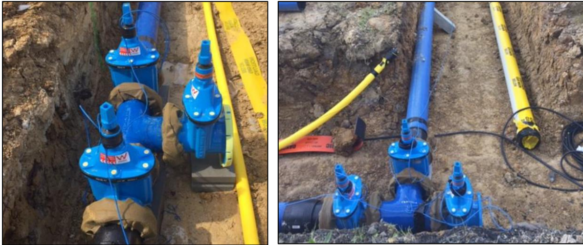
Figure 4: Examples of isolation valves installed on the principal water main at a road crossing.
