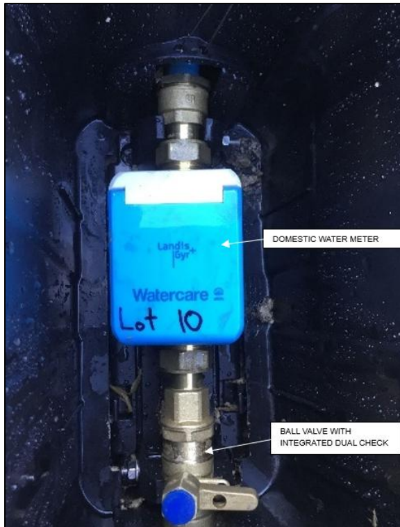
Figure 22: 2) Installed single domestic water meter.
