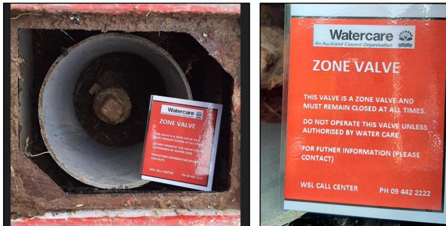
Figure 8: Example of installed zone valves and valve tag.
