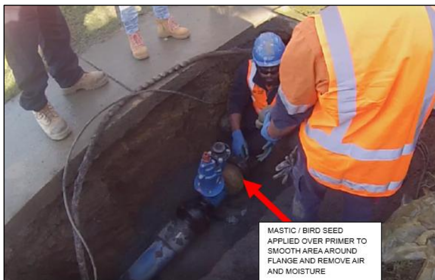
Figure 33: Application of mastic (Part2)
