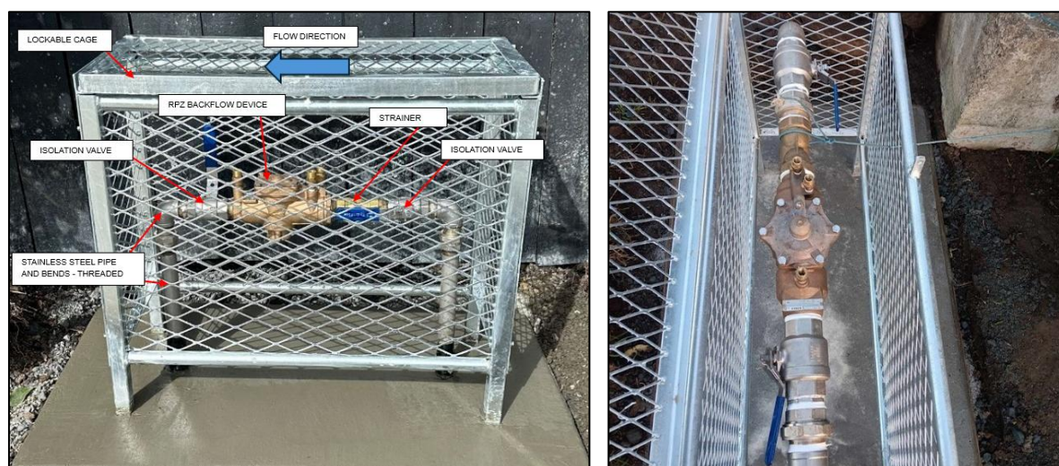
Figure 23: Installed backflow prevention device for a high-hazard location.
