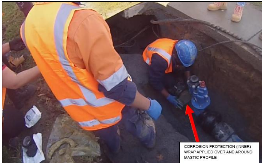
Figure 34: Application of corrosion protection tape (Part3)
