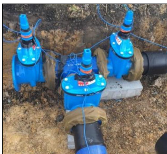
Figure 18: Installed sluice (gate) valves prior to reinstatement.
