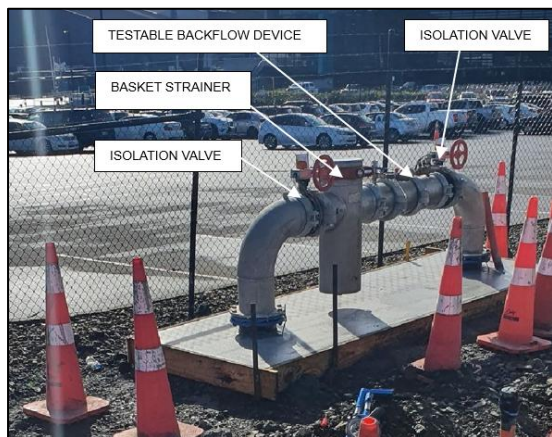
Figure 26: Example of a testable backflow device and endorsed basket strainer (RPZ aboveground).
