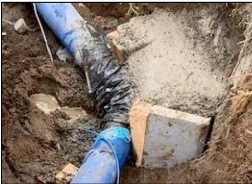
Figure 11: Example showing PE sleeving around the pipe.
