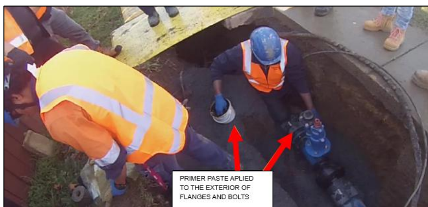
Figure 32: Application of primer (Part1)
