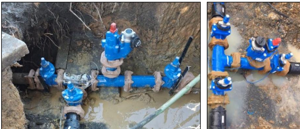
Figure 5: Examples of isolation valves including a hydrant installed at a road crossing to accommodate flushing the line.
