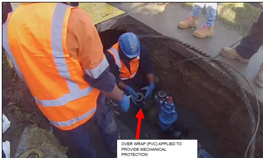
Figure 35: Application of overwrap PVC tape (Part4)
