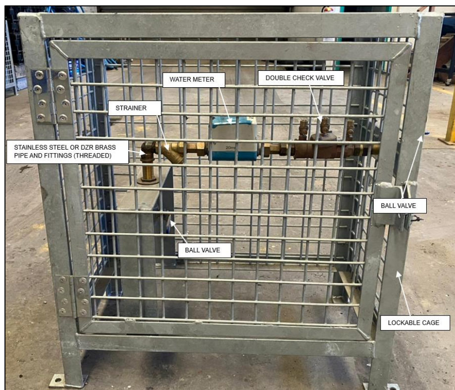
Figure 29: Assembled 20mm diameter temporary construction water meter.
