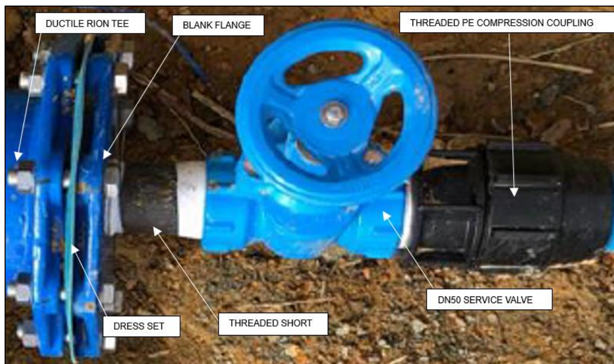
Figure 7: Installed example of a DN50 rider main connection from a 100mm principal main.
