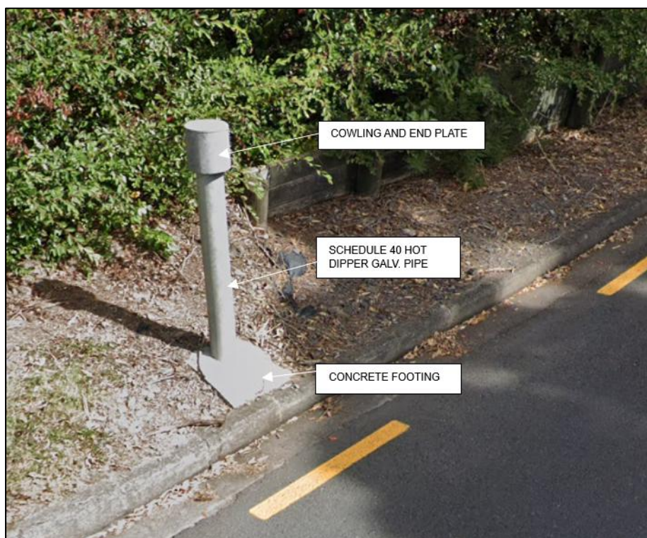
Figure 20: Installed air vent, from air valve chamber.
