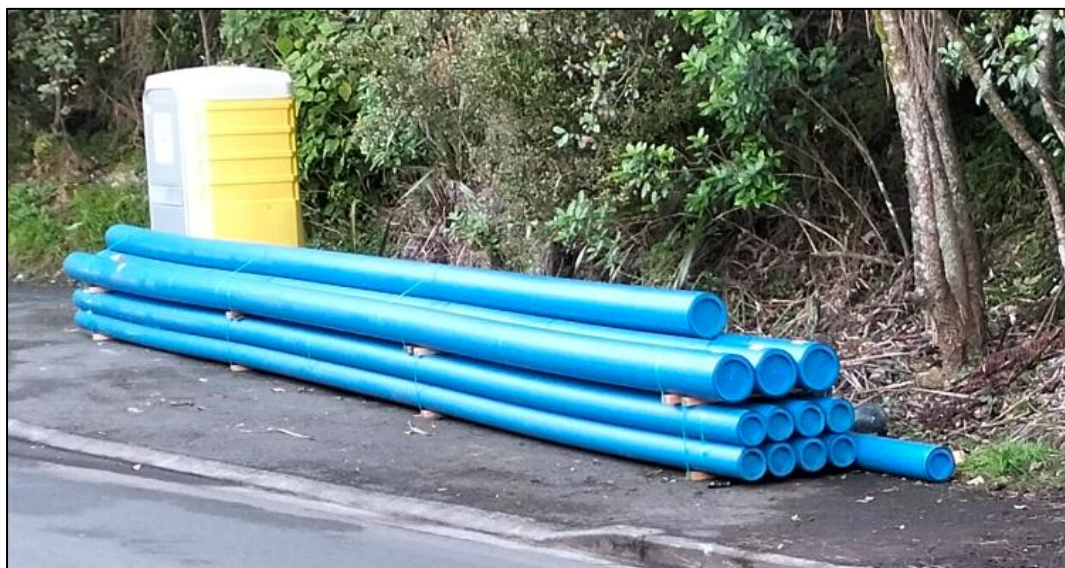
Figure 1: Example of materials stored on-site with appropriate capping.
