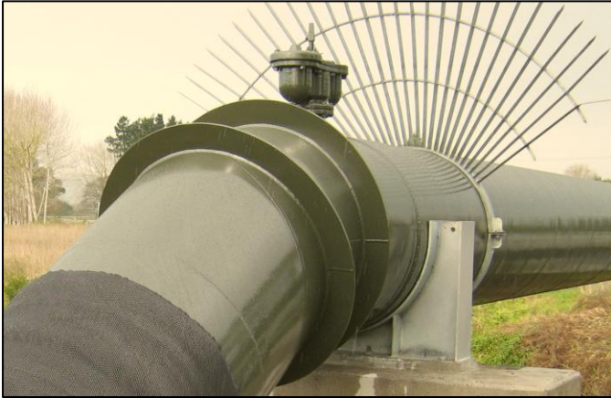
Figure 4.1: Example of a standalone pipe bridge located in natural environment.
