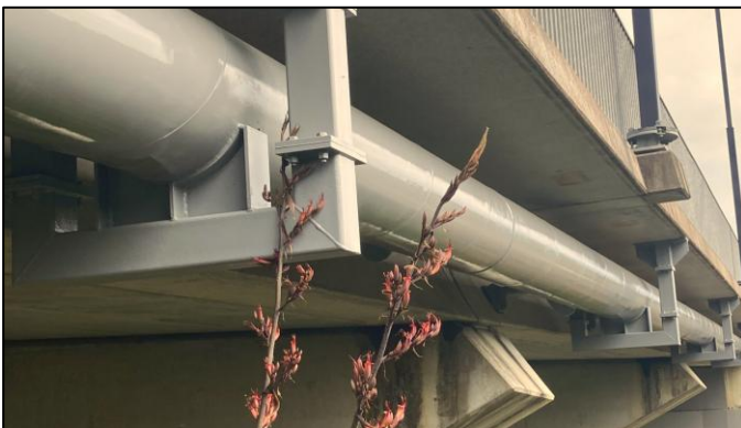
Figure 4.2: Example of a pipe bridge incorporated in a road crossing (colour: BS5252: 16 A07)
