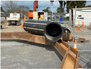
Archboyd Avenue Driveway sheet pile and bulk cut to working
